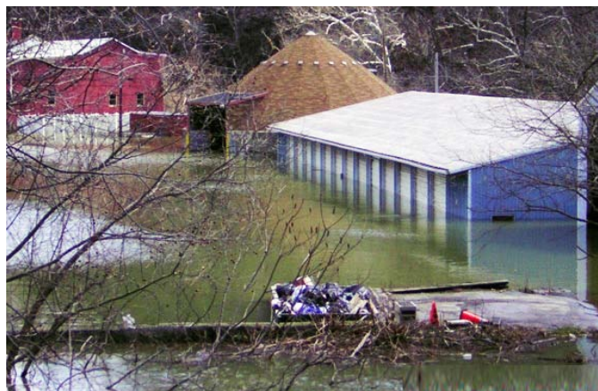
Damage from Hurricane Ivan (2004). Photos courtesy of City of Easton Fire Department
